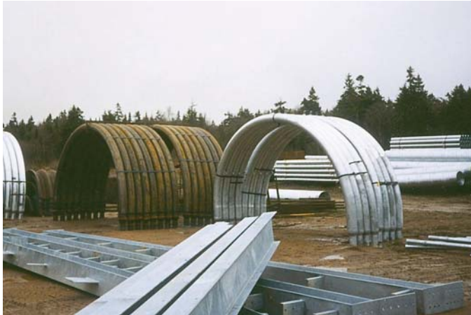
Pre and post-galvanized post tensioning return loops for the Confederation Bridge
